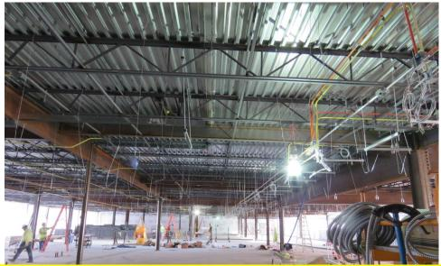
If the specifications indicate that the attachment to the metal deck is not acceptable, we might want to review and verify with the structural engineer of record.
