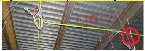
If the attachment is found to be acceptable, it is best NOT to attach to the <u>low</u> part of the flute. Condensation might form below the roofing and create a hole in the <u>low</u> part of the <u>flute</u> might introduce moisture into the building.
